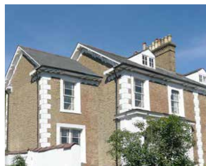
Community: Best practice photograph A similar architectural approach is continued in this side extension by Sam Causer
